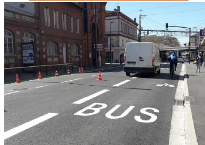
COULOIR BUS FBG BONNEFOY
